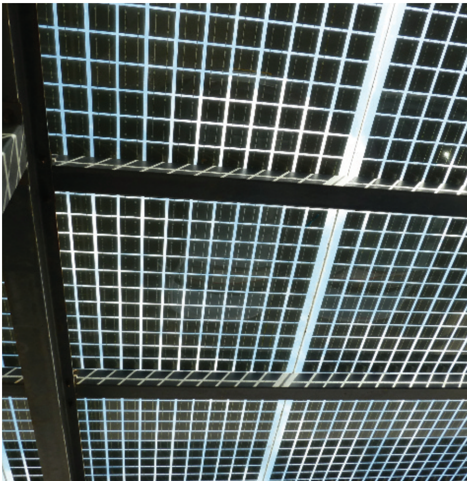
Picture 1 – rows of solar cells provide shade whilst generating electricity at Solar Capture Technologies, Blythe.
